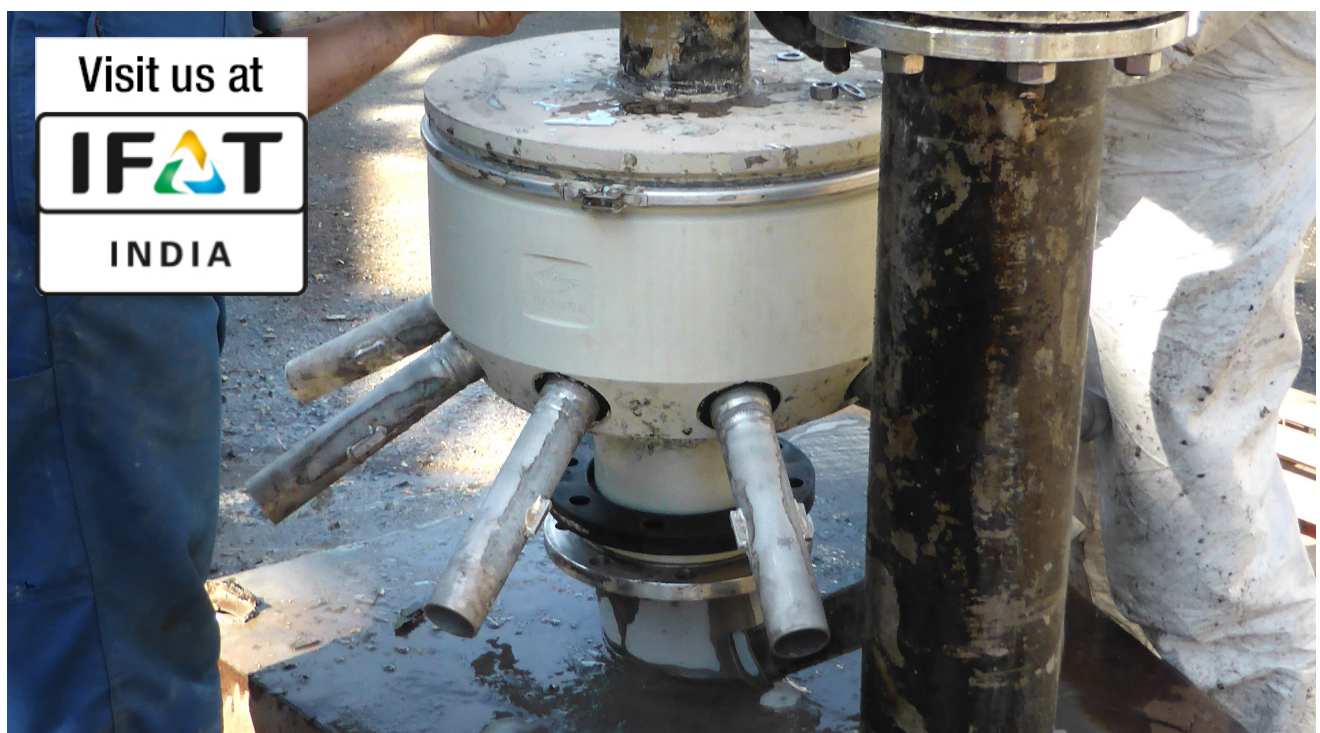
Removing one of the bodies on the 8-jet waste water aeration ejectors – the stainless steel ejector arms are easy to see
